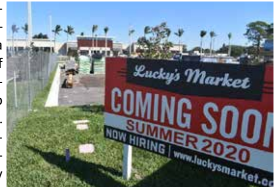
Lucky's Market signs are remain up — but construction appears to have stopped. (Aldi's may take the space)
